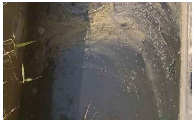
Fig 3: Condition of the observed drain.
